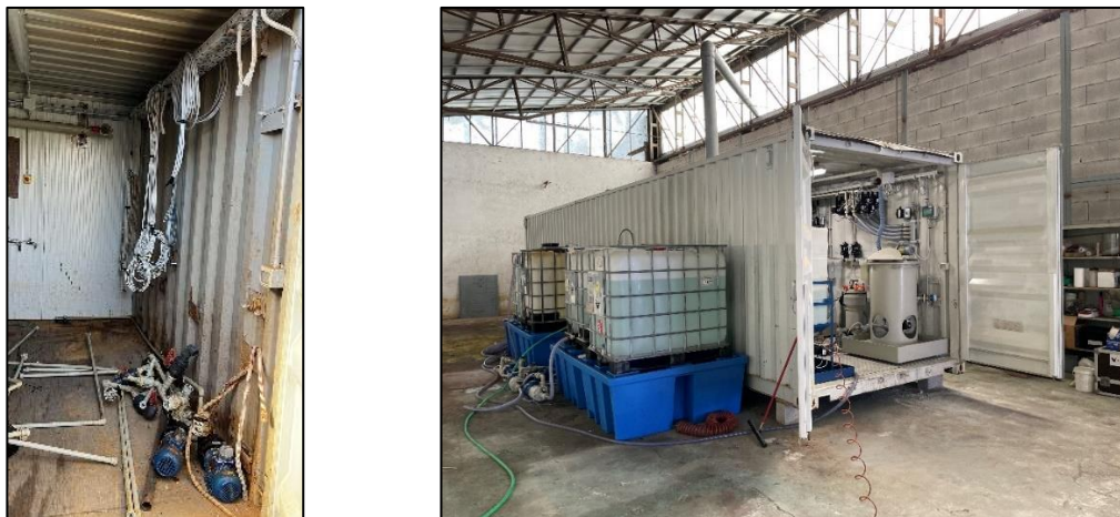
Figure 10: Picture of the plant during and after the reconfiguration works.
